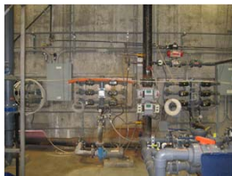
Side view of whey digester showing plumbing, pumps and controls
