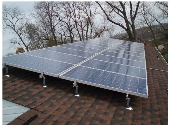
Roof Mounted PV Panels use specially designed hardware to attach to the roof without compromising water tightness.
